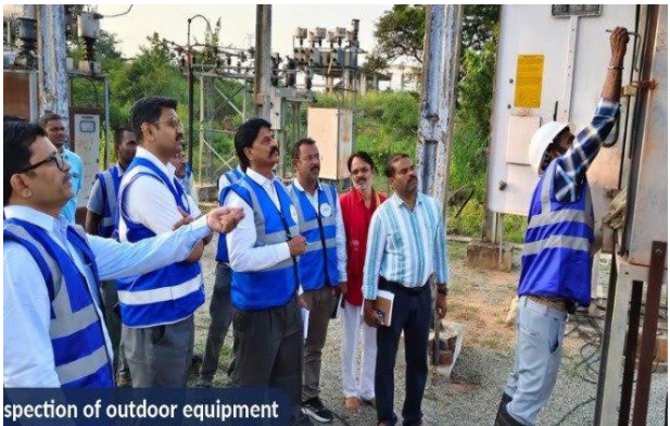
Inspection of outdoor equipment
